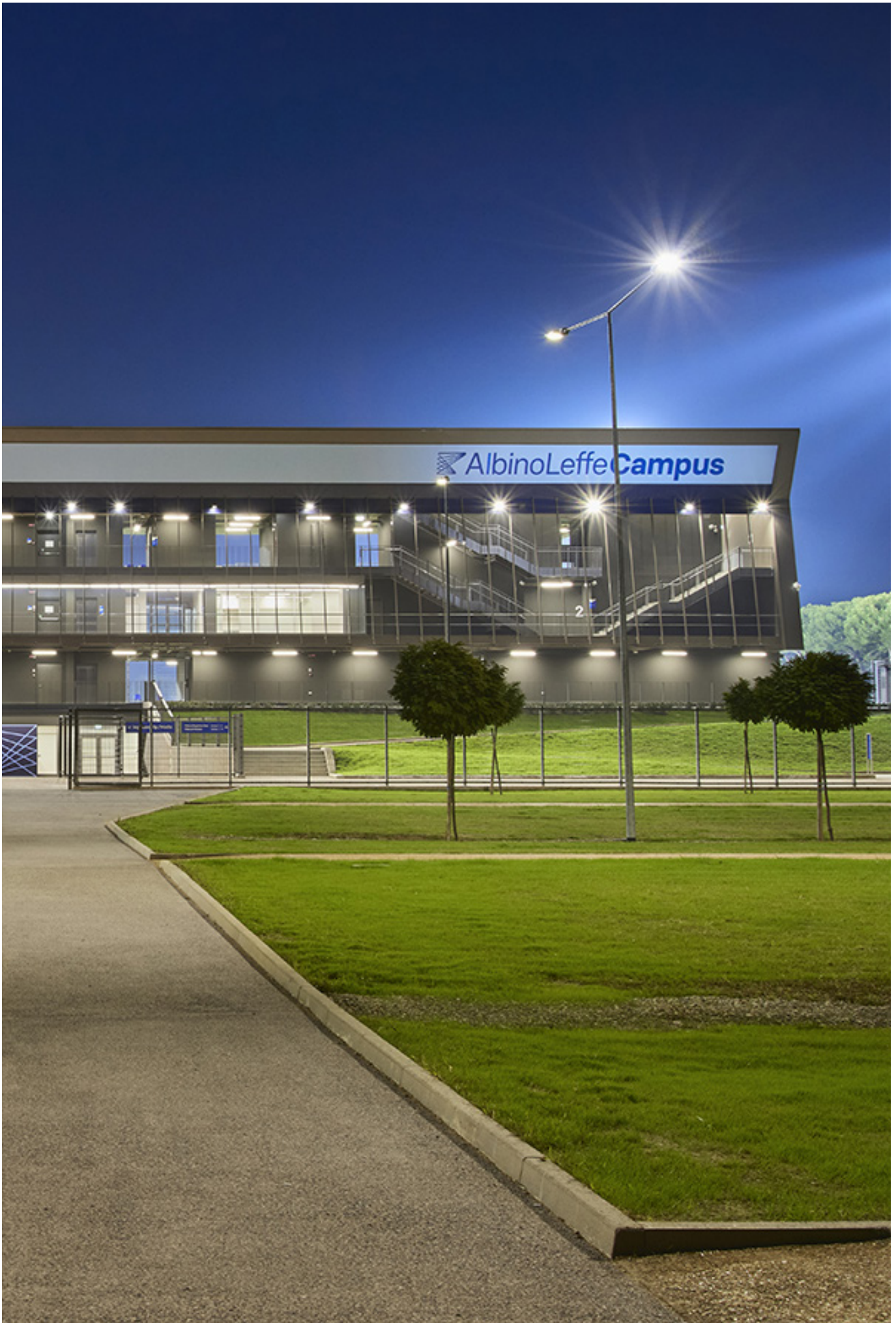
Albinoleffe stadium - Zanica - Italy
