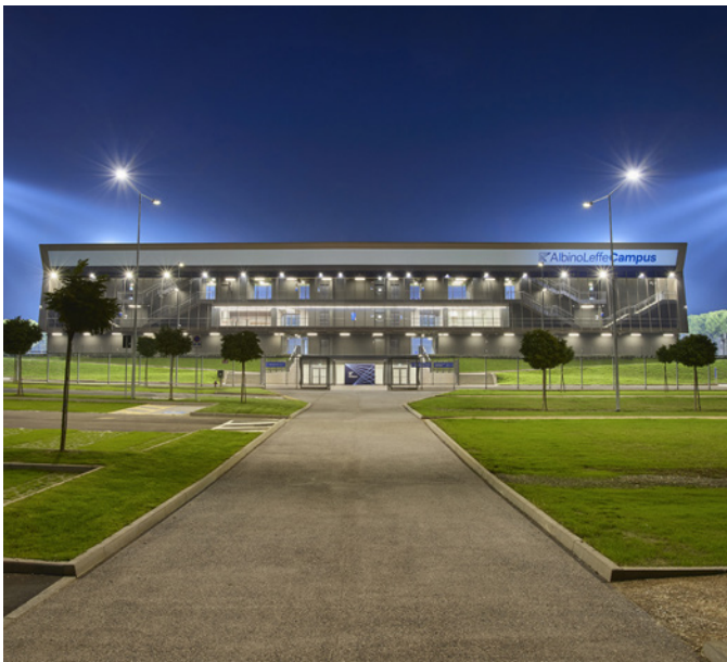
Albinoleffe stadium - Zanica - Italy
