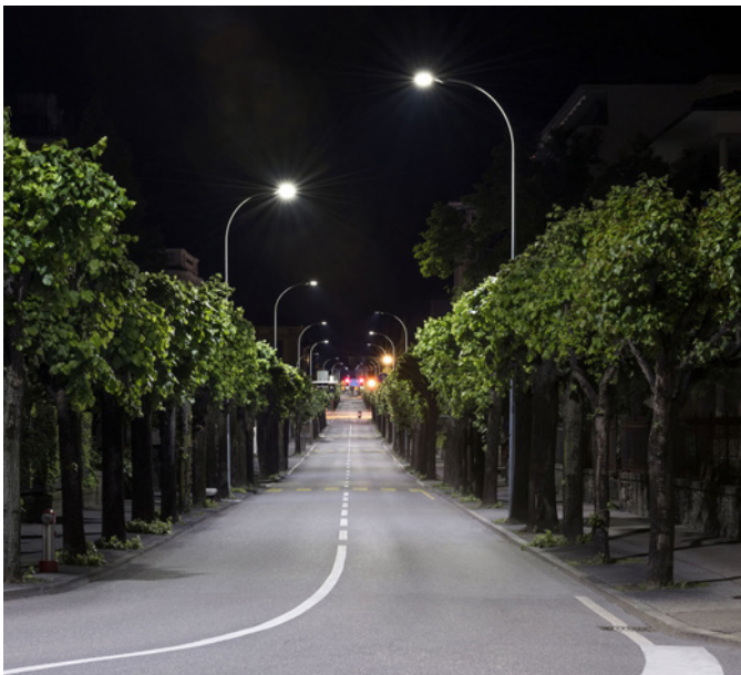
Municipality - Bellinzona - Switzerland
