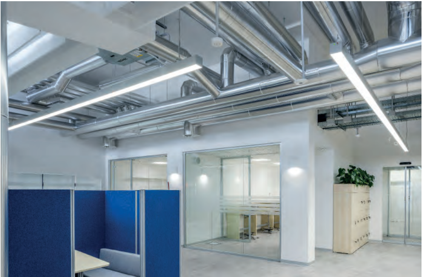
Offices comprensorio Olivetti | Naples | Italy
