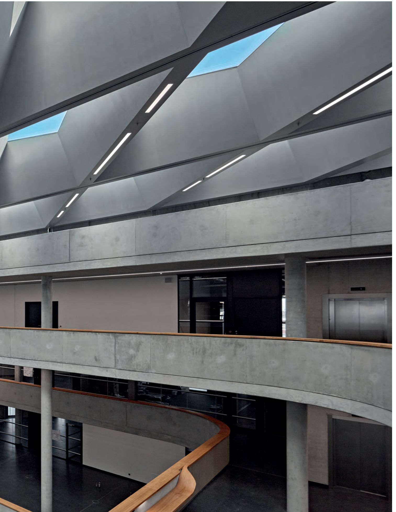
Zalando headquarters | Berlin | Germany
