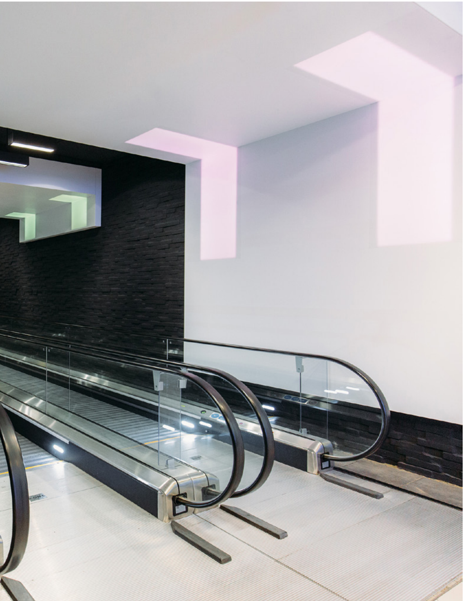
Verbindingstunnel van heekgarage | Enschede | Netherlands
