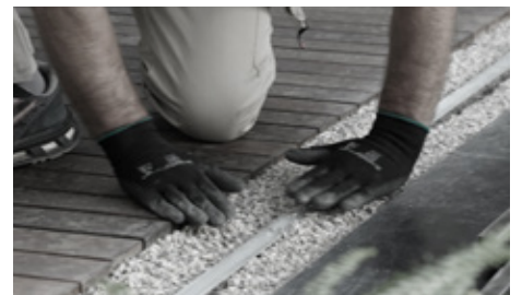
For outdoor applications, provide drainage gravel for at least 300 mm additional to the appliance or a suitable drainage system
