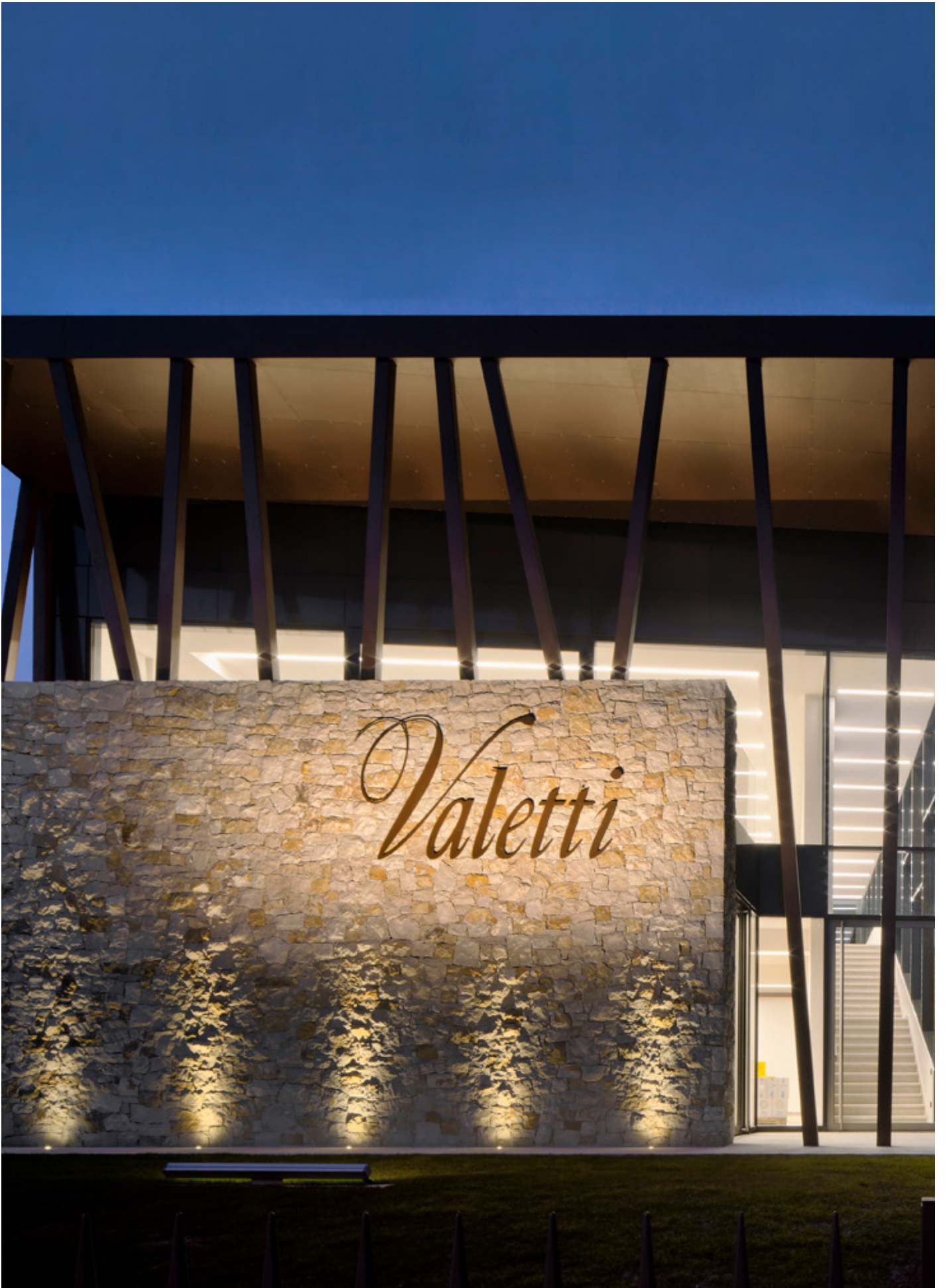
Valetti winery | Bardolino | Italy
