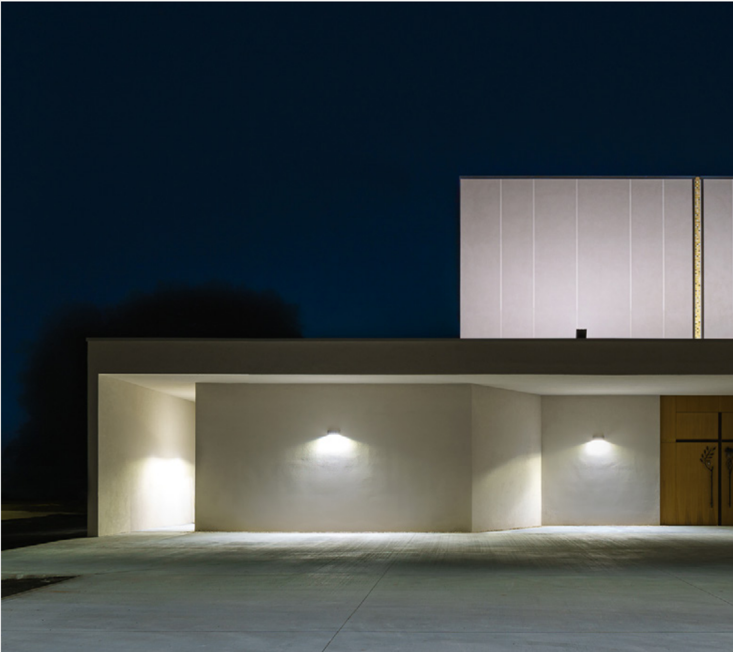
Parish Complex | Varignano - Viareggio | Italy
