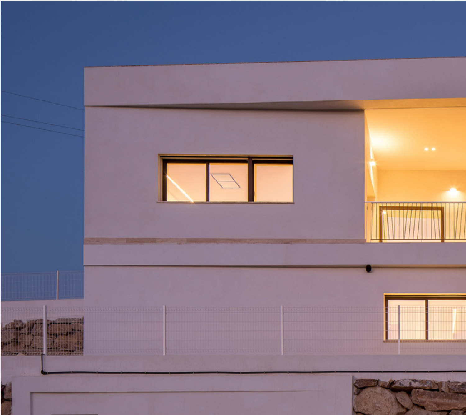
House in Albánchez | Almería | Spain
