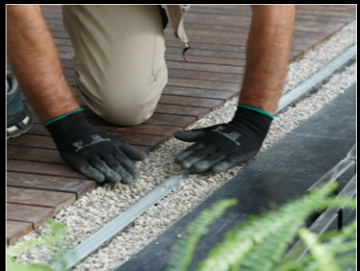
For outdoor applications, provide the appliance with drainage gravel for at least an additional 11.8 Inches or an adequate drainage system.
